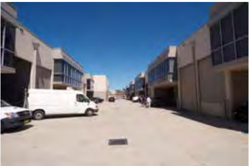
11 Victoria Road Industrial Estate
